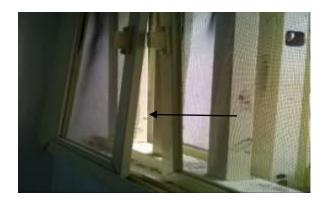
Plate 8: Window net frame not properly aligned with vertical opening- urban.
