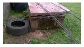
Plate 9: Septic tank with the upper closure slab not properly aligned nor sealed, with openings enough for mosquitoes to hide and rest inside tank-urban.
