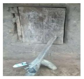
Plate 1: Window not properly aligned and cannot be shut-rural area
